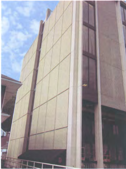
Existing Precast Concrete Panels
