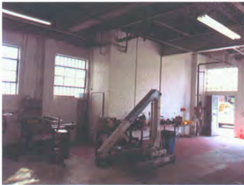
Diesel Shop Interior
