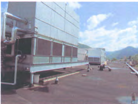
New Rooftop Mechanical Equipment
